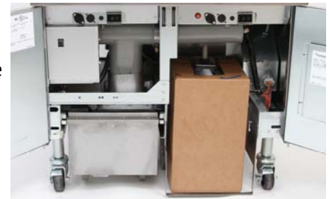
Figure 1: The fryer prior to the install is show above. The sensor mounts on the channel behind the center upright. The pre-filter mounts above the filter pan pickup .
